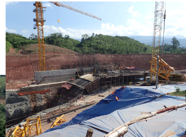
Sediment management during construction
