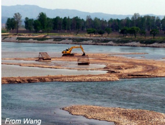
Dredging of bedload Yangtze, China
