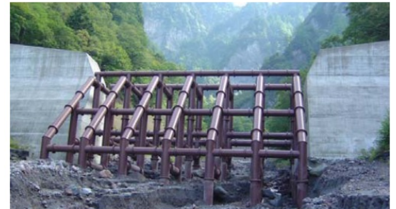
Check dams on tributary inflows
