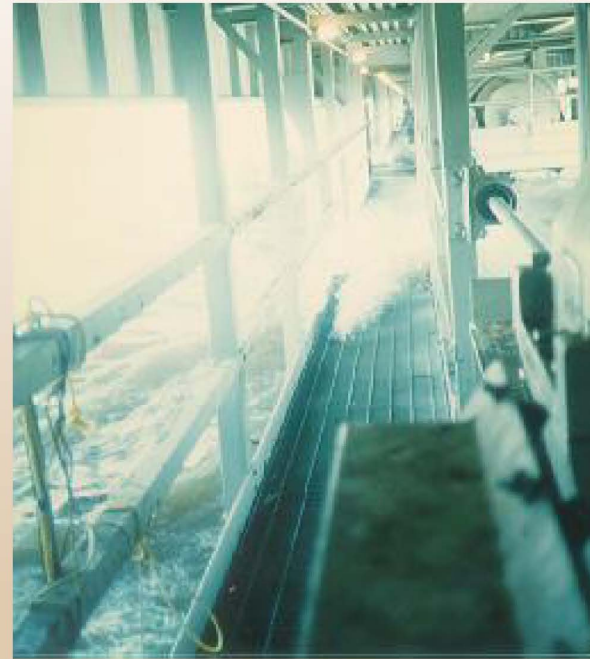
Catwalk almost inundated during flood – gates must be operated from catwalk
