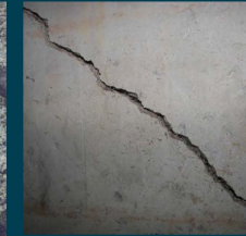
Diagonal Cracks
