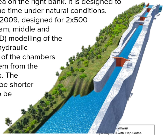
Figure 3-4 The two-step navigation lock system.
